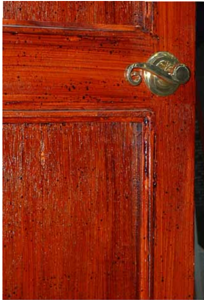
THIS CLOSE-UP SHOWS A SECTION OF A PANEL DOOR PAINTED WITH A BRIGHT ORANGE UNDERCOAT, AND A VAN DYKE BROWN GLAZE.
