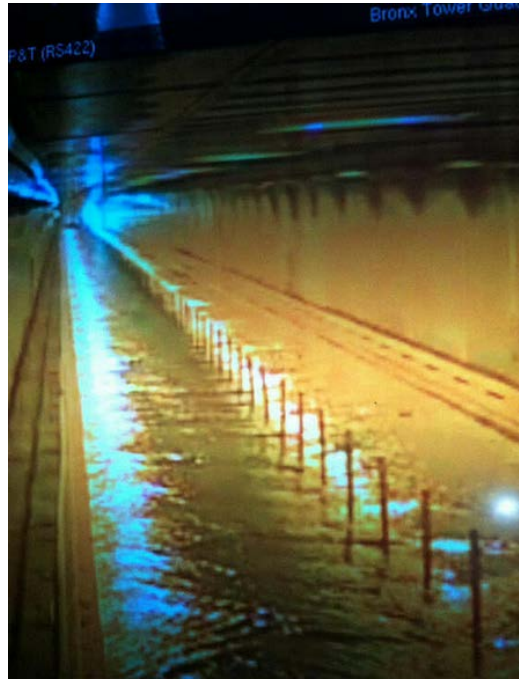
Figure 31. Flooding in the Brooklyn-Battery Tunnel (New York Times 2012).
