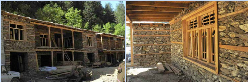
Figure 17 Construction using locally adapted techniques (Malan 2012).
